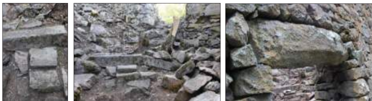
Fig. 52,53. Entrance from W. Stone steps.
