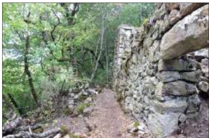
Fig. 45. N wall from outside. View from NW.
