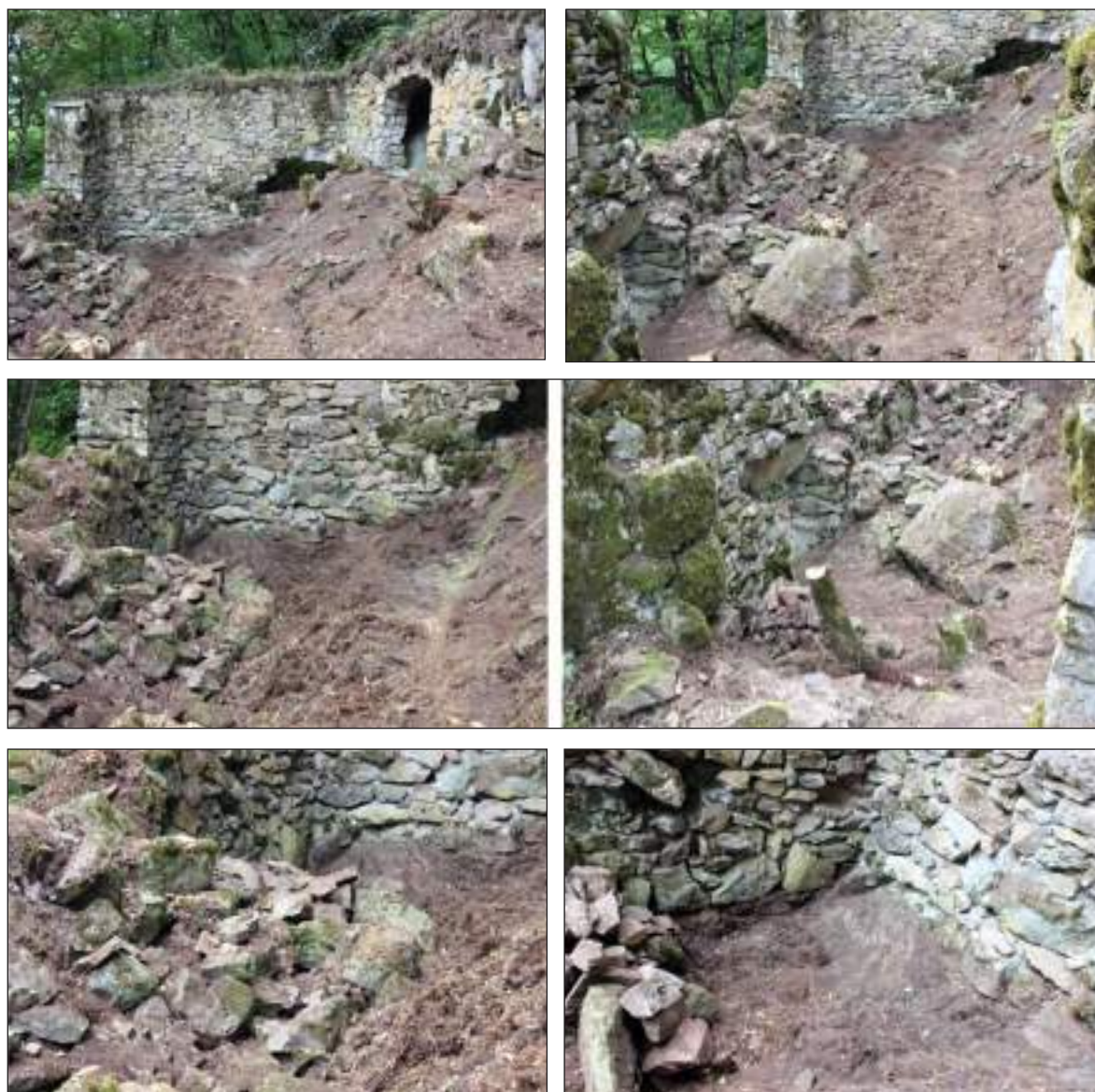
Fig. 55-60. The refectory at various stages of work. Photo by T. Bibiluri
