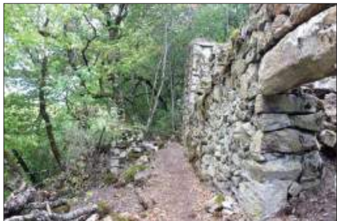
Fig. 45. N wall from outside. View from NW.
