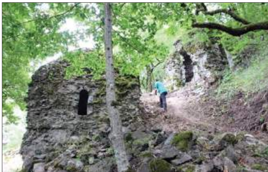
Fig. 39. Road between III and IV terraces
