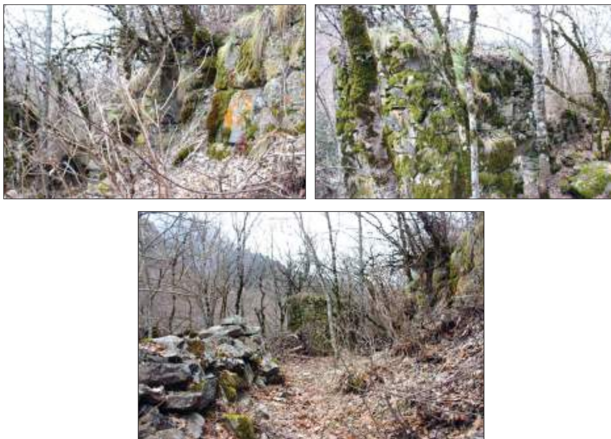
Fig. 46-48. The refectory before works. Photo by T. Bibiluri
